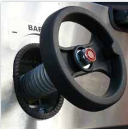
Infinitely adjustable pressure regulator mounted at a least frost-sensitive position
