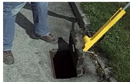
5: Rotate cover to the open position
